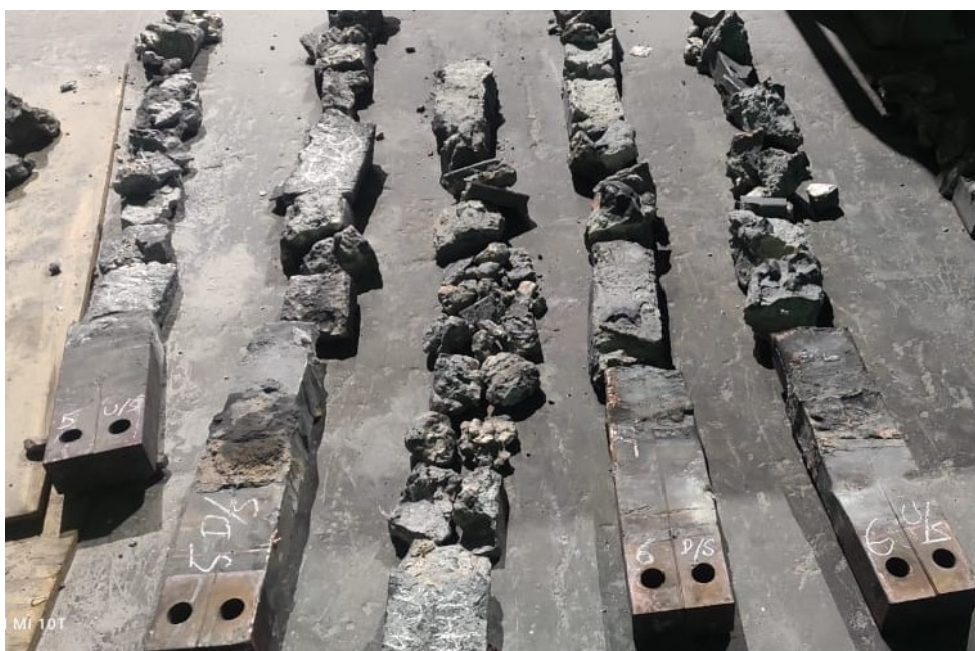
Figure 18. Cu bars of low current pickup after being taken out from the cathode blocks.
